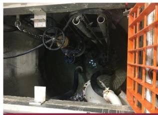
GPM-Eliminator Submersible Pumps in Water Treatment Process
